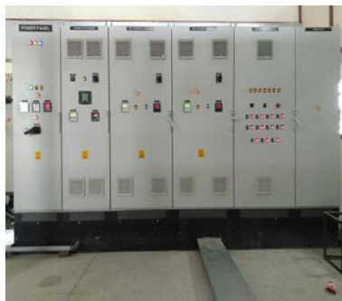
Power panel for Industrial grade Autoclave
