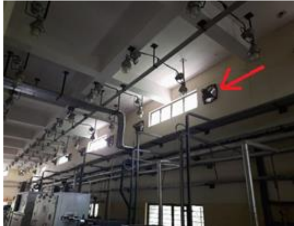
Figure 3 : Fiber spinning area Exhaust fan location
