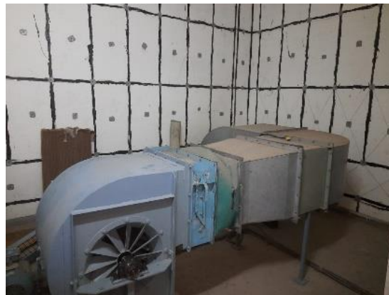
Figure B1 : Existing HVAC room for proposed clean air supply room
