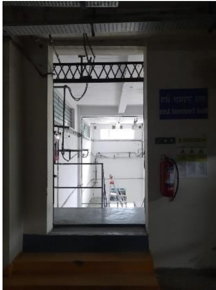
Figure 1 : Picture of Fiber spinning area (Exit door):
