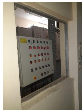
Figure 4 : Motor ON/OFF panel isolation in fiber spinning area
