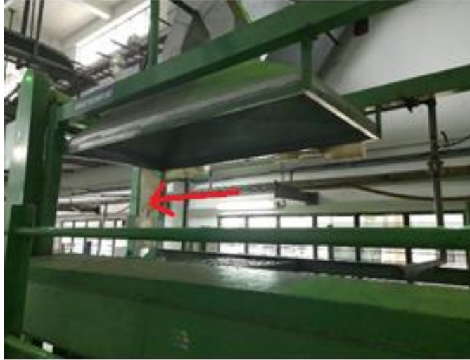
Figure 5 : Surface treatment unit
