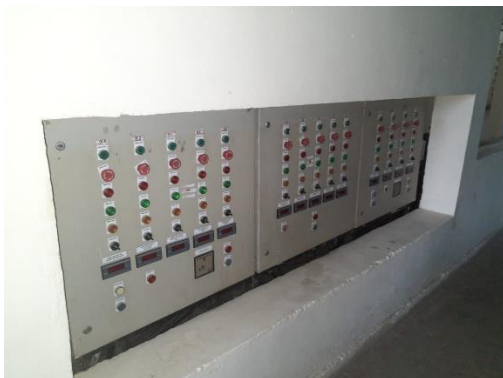
Figure 4 : Motor ON/OFF panel isolation in fiber spinning area
