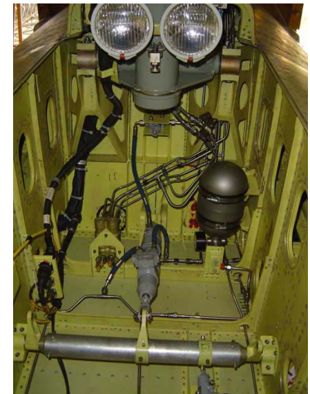
Hydraulic installation in NLG bay
