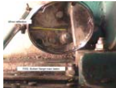
A fatigue crack also initiated from the same bolt hole on the starboard side.
