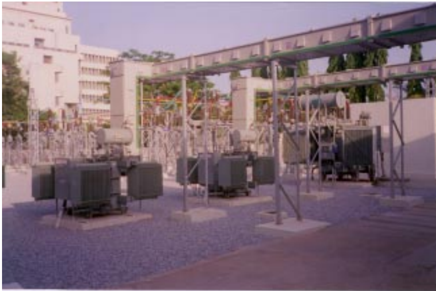
↑ Figure 12: The new 66 kV 10 MVA electrical substation at the Kodihalli campus significantly enhances NAL's comfort factor vis-à-vis electrical power supply.
