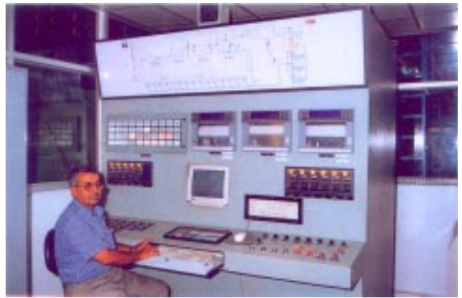
↑ Figure 5: The instrumentation system of the 4m x 8m autoclave recently handed over to NAL.
