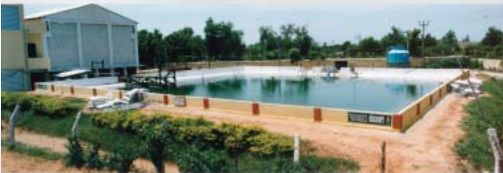
The 500m 2 experimental salt gradient solar pond.
