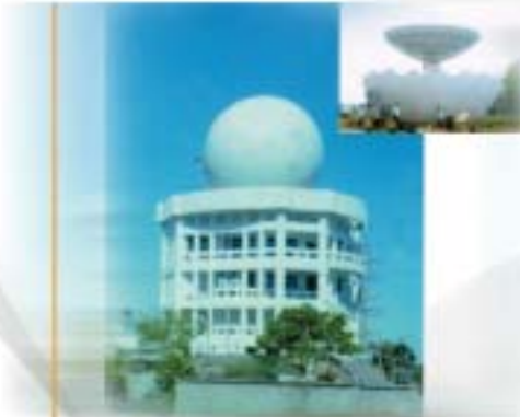
12.88 DWR radome to protect cyclone warning radar.
