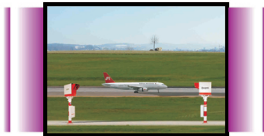
DRISHTI is installed at the cochin and Lucknow airports
