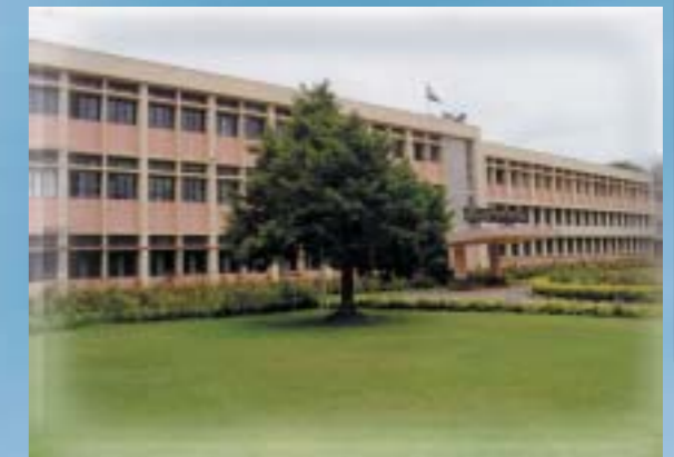
NAL's main building.
