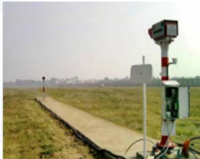
Drishti installed at Indira Gandhi International Airport
